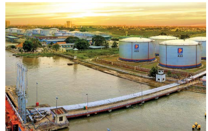
Petrolimex is energising the economy with key power projects.
